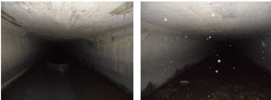
Figura 24. Box Culvert La Castellana, vista interior
