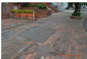
**Figura No. 29 Adoquín en arcilla**
